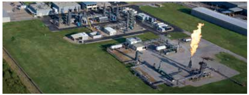
RESEARCH AND DEVELOPMENT TEST CENTER
