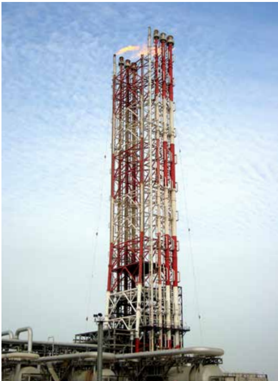
MULTI-FLARE TIP DEMOUNTABLE FLARE STRUCTURE
