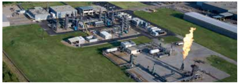
RESEARCH AND DEVELOPMENT TEST CENTER
